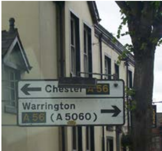
Figure 11-1 Sign obscured by lighting unit
